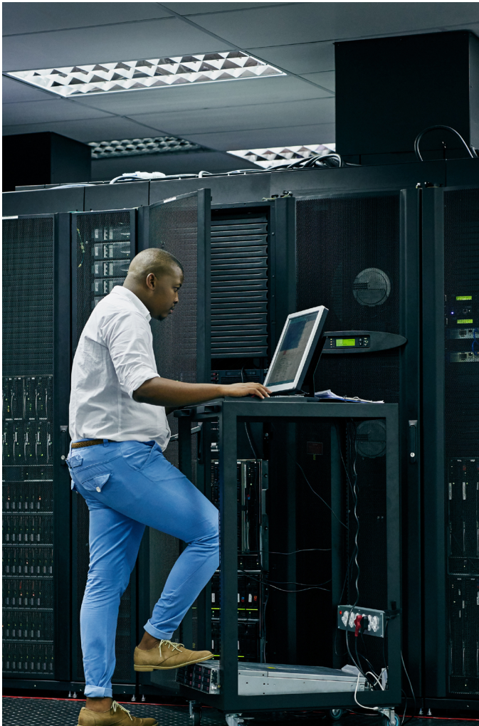
MemberClicks has streamlined its order-to-cash cycle through integrating Sage Intacct with its Salesforce CRM application.
